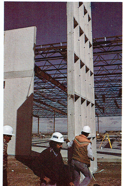
Waffle-Crete panel 28 ft. tall produced for warehouse project.
